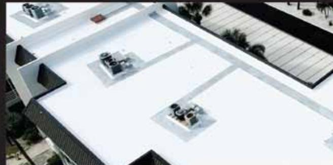
Uniflex® Premium Elastomeric White Finish Coat is formulated using a 100% acrylic polymer that provides outstanding weathering and superior reflectivity properties.
